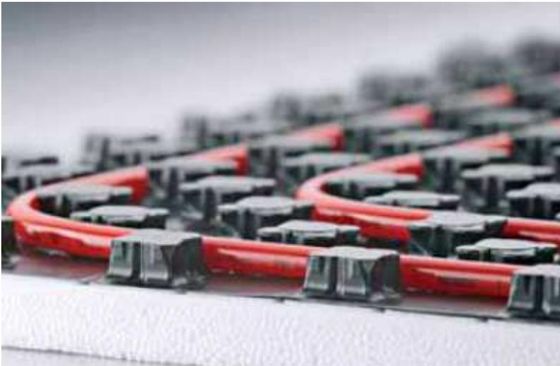
**Figure 5 & 6: The thermal distribution system based on the heating/cooling floor**
